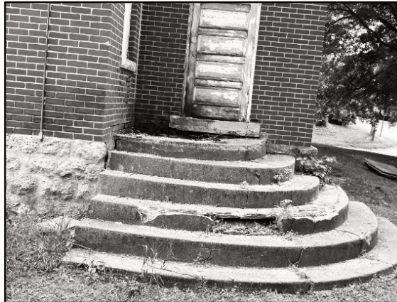
Steps leading to the Elysian school's southwest entrance is just one component of LCHS's efforts to restore the historic structure.
